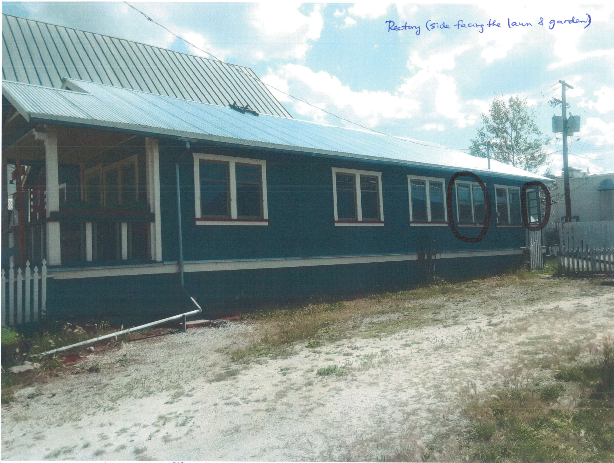
Keep first 3 windows to match original building. Remove 2 circled windows in the extension of the building.
