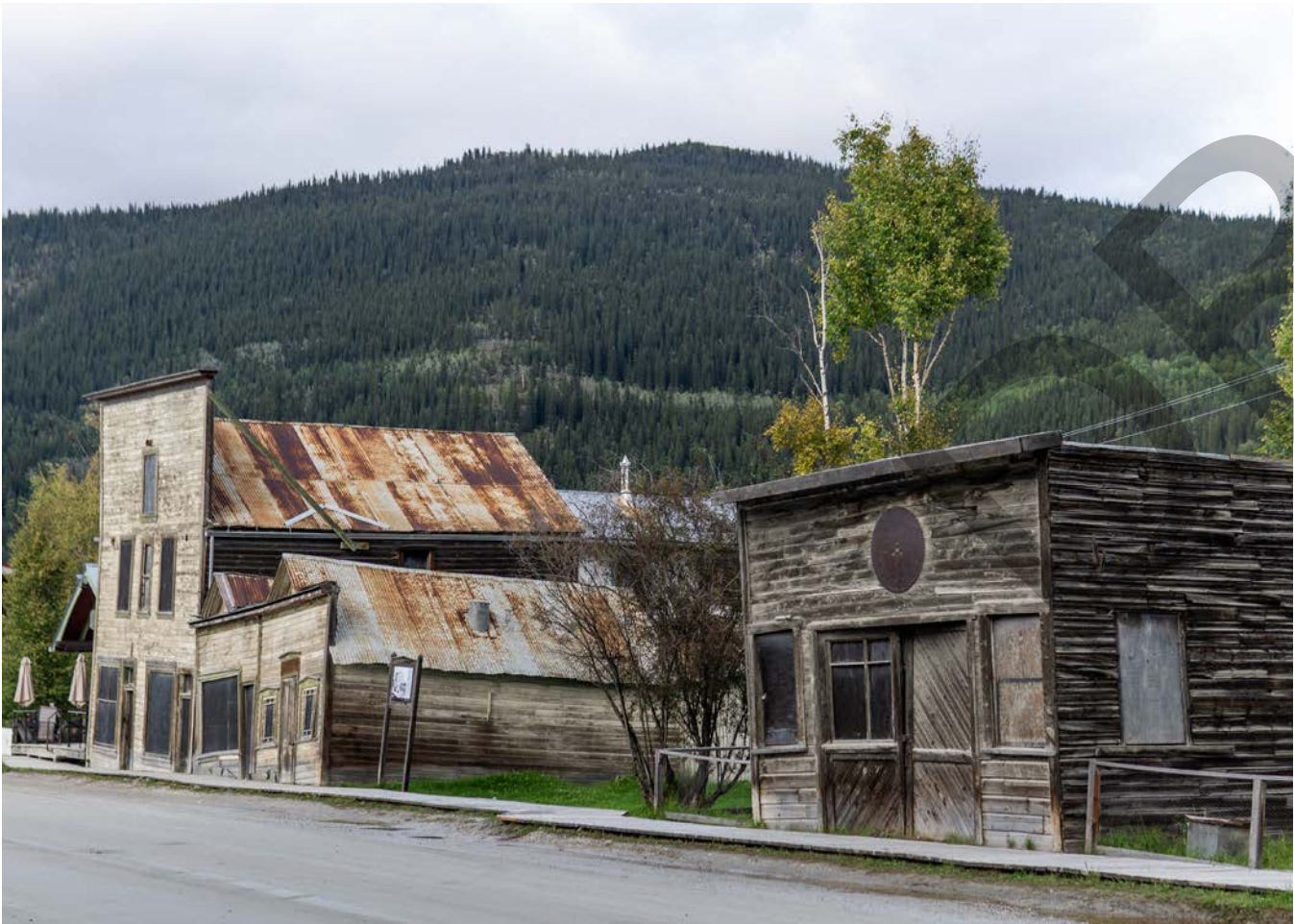
Figure 5: Third Avenue Hotel Complex, colloquially known as the “kissing buildings” as the building is slanting due to permafrost degradation and has been stabilized by Parks Canada
