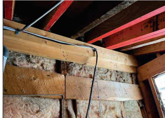
Figure 2-12 Lean-to-Roof Connection with the Main "Hall"
