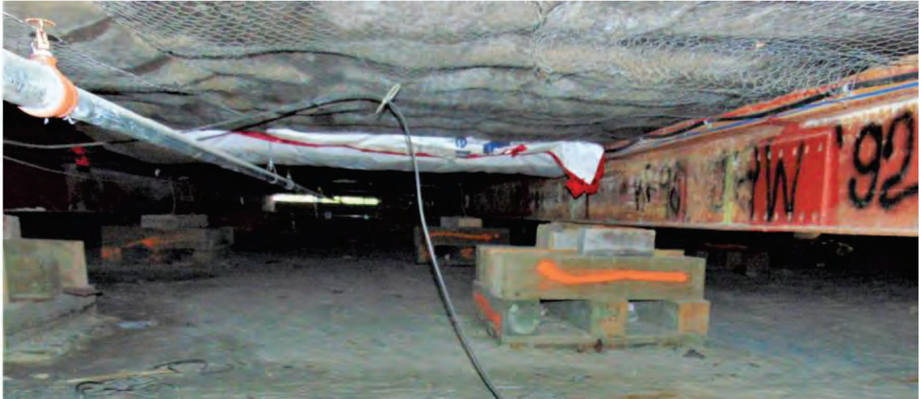
Figure 2-18 Steel Beams without Lateral Support at Support Locations
