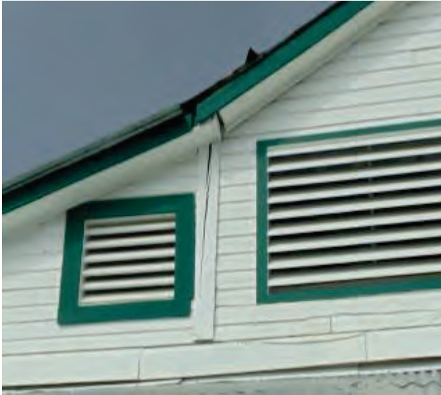
Figure 2-11 Two Photos of Separation between South Lean-to and Main "Hall"
