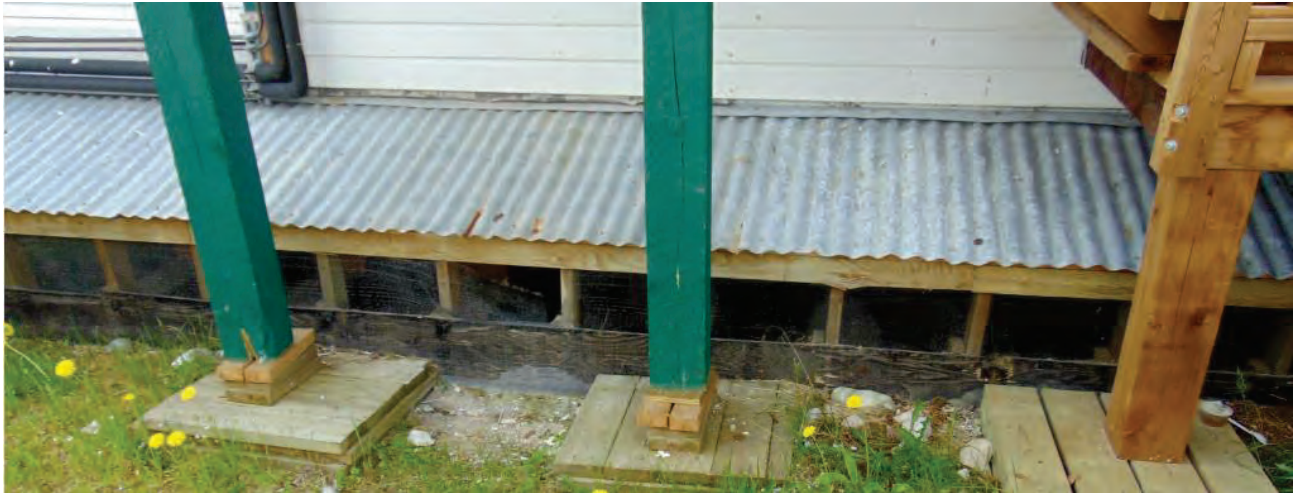
Figure 2-1 Poor Lateral Support at the Base of Fire Escape Columns
