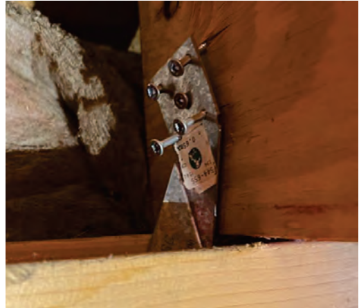
Figure 2-14 Rafter Cleat Pull Outs
