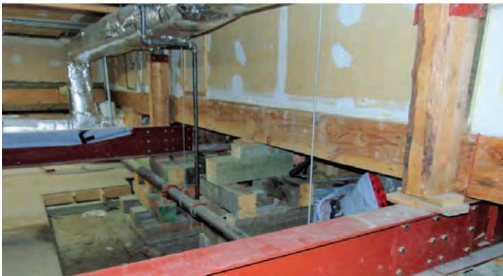
Figure 2-19 Props to Back of Stage as Seen from Basement
