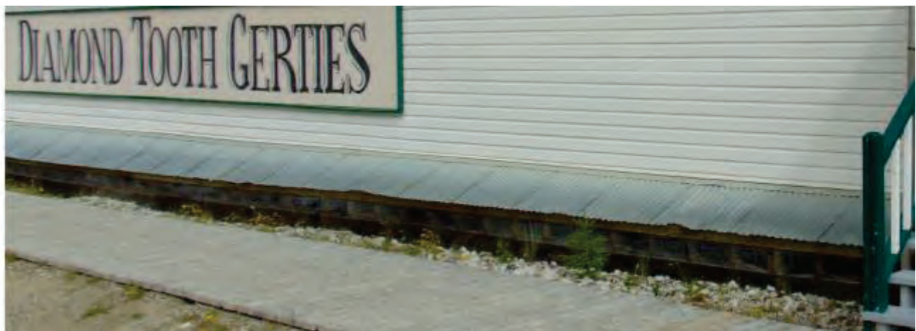
Figure 2-2 Offset Crawlspace Wall Permitting Large Amount of Air Movement
