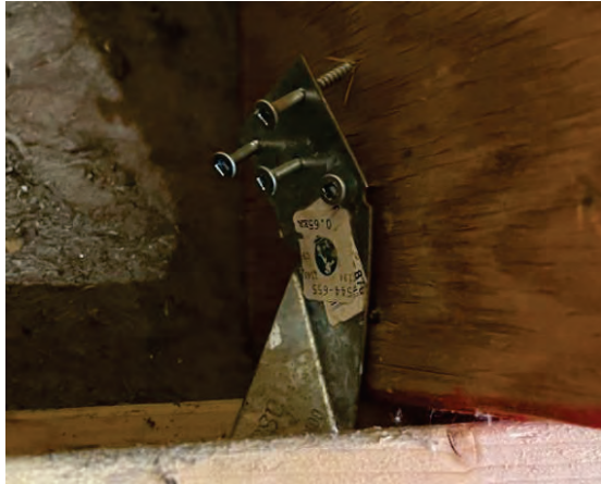
Figure 2-14 Rafter Cleat Pull Outs
