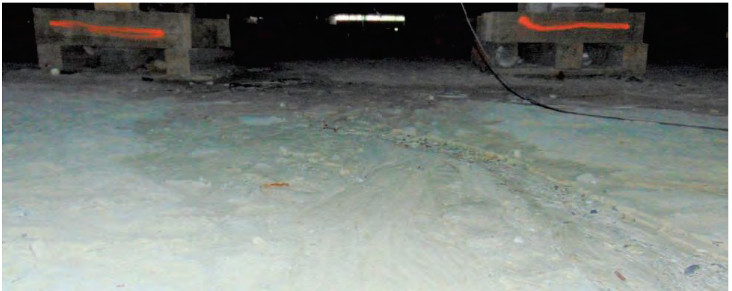
Figure 2-4 Crawlspace Surface Showing Meltwater Running Towards Northeast
