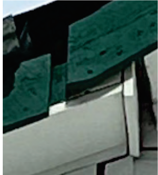
Figure 2-11 Two Photos of Separation between South Lean-to and Main "Hall"
