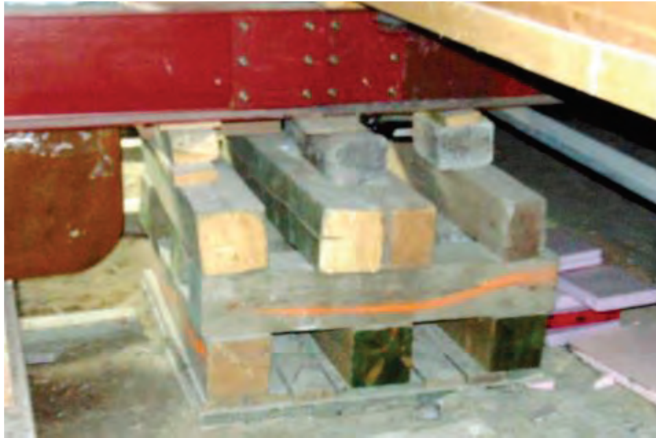
Figure 2-17 Typical Cribbing Showing Shims Under Steel Beams
