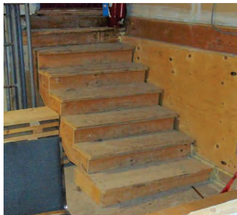
Figure 1-1 Under Staircase, Note Extension at Base
