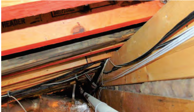
Figure 2-12 Lean-to-Roof Connection with the Main "Hall"
