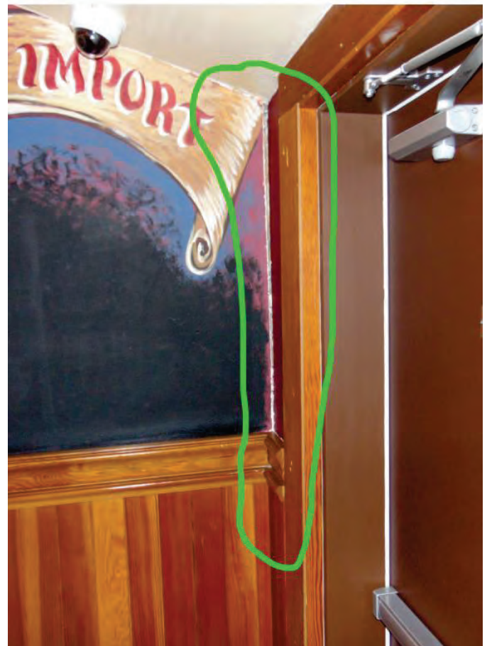
Figure 2-6 Separation of South Wall
