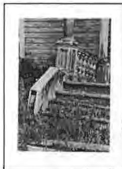
8: Veranda column and balusters
