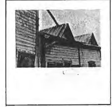
5: Entablature with exposed gable
