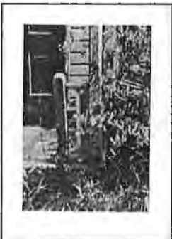
6: Veranda column and balusters
