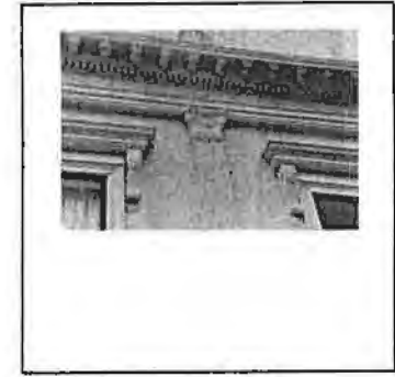
7: Pressed tin column and entablature
