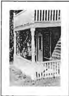
1: Veranda and balcony
