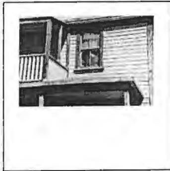
1: Typical residential window
