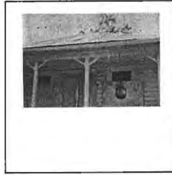
2: Veranda - column treatment - hip roof
